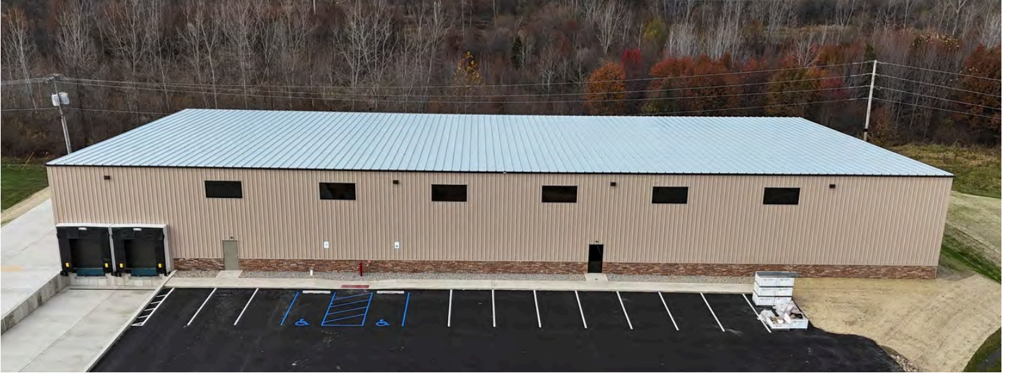
Spec Building, Arden Drive, Fort Wayne
